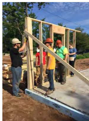
Putting up the first wall
